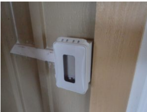
Installed Surface Mount Box (with window!)
